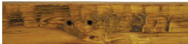
Hand Adzed Beams
